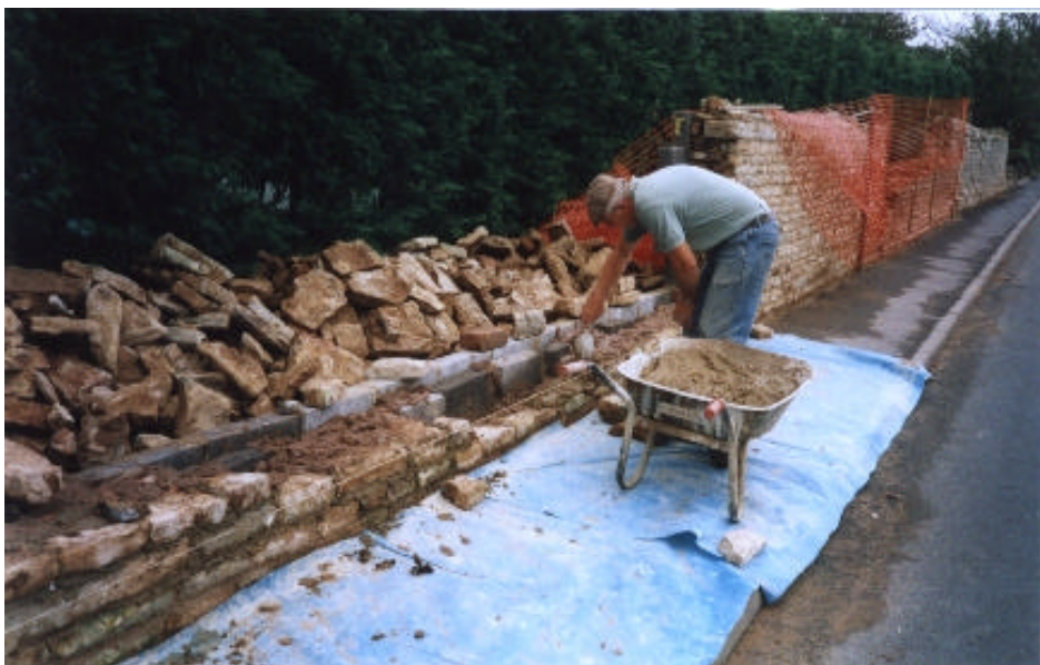
Manor House wall under reconstruction
