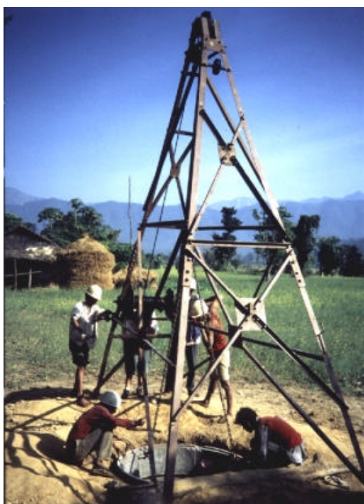
Drilling a new Village well
